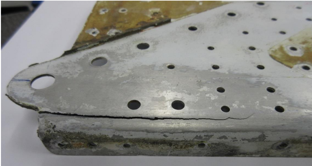
Figure 1 – Crack in Front Spar
